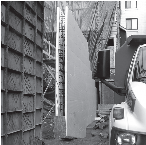
Figure 5.9: Insulating concrete forms (ICFs) consist of rigid insulation tied together with metal ribs (photo by the author)
