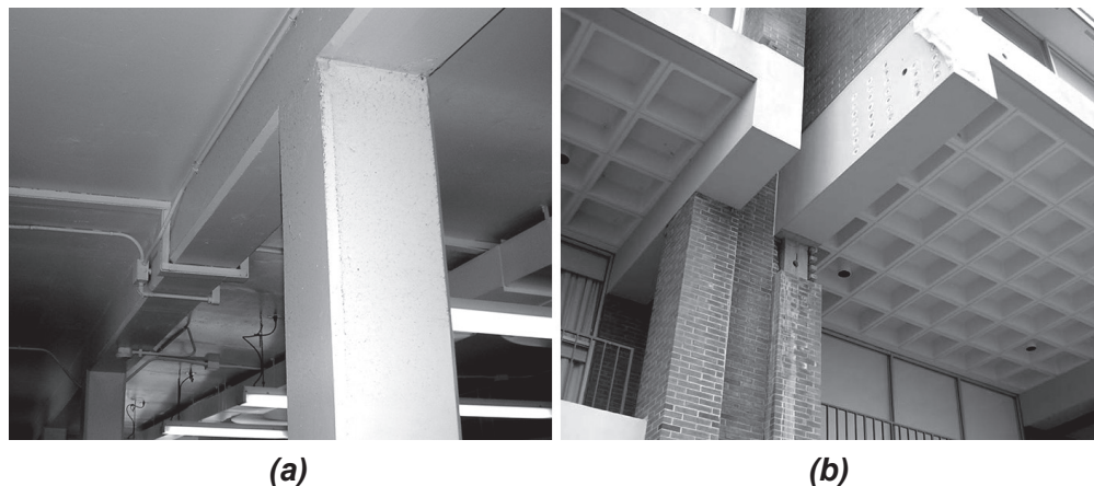
Figure 5.15: (a) One-way slabs span directly between reinforced concrete girders supported on square columns, Teagle Hall, Cornell University, photo by the author; (b) two-way grid slabs are supported on cantilevered girders, Robert Purcell Community Center, Cornell University, photo by the author
