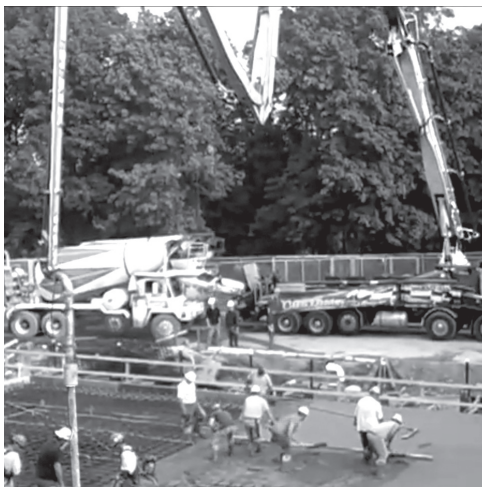
Figure 5.12: Concrete for a slab is pumped from a remote vehicle
