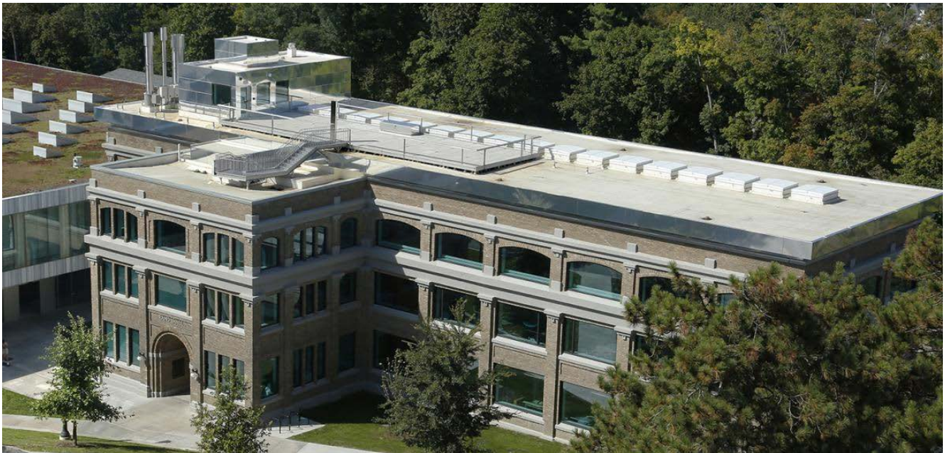
The accessible roof has a structurally reinforced deck to host full-scale experimental pavilions that will be designed and fabricated by Cornell faculty and students. Temporary and speculative, these constructions will anchor the site with rooftop testimonials to ongoing research in architecture and the built environment.
