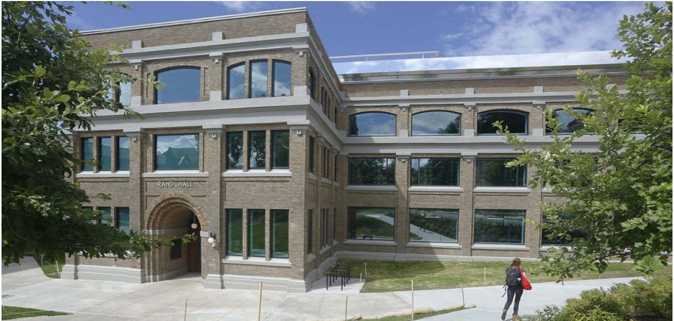
The entire building envelope was remediated during construction, including thermal insulation and double-glazed windows that significantly improved the energy performance of Rand Hall.
