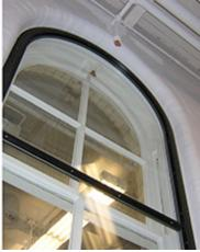
Figure 3. (Left image) Non-fire-rated window violates the fire barrier between Rand and Milstein Halls: Cornell never completed the fire barrier between Rand and Milstein Hall. Not only does it not have a 1-hr rating as was required at the time, portions still do not have any fire-resistive rating at all.
