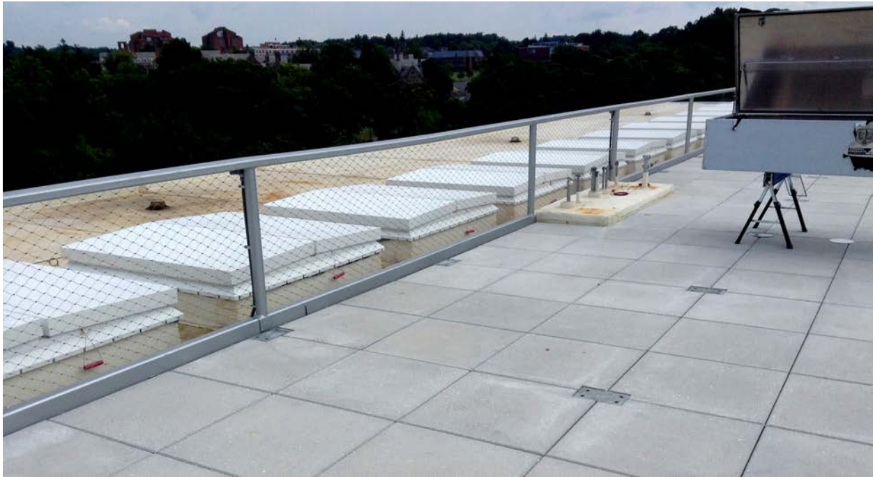
Appendix Figure 1.3. Smoke hatches form the northern boundary of the roof-top art gallery assembly space.
