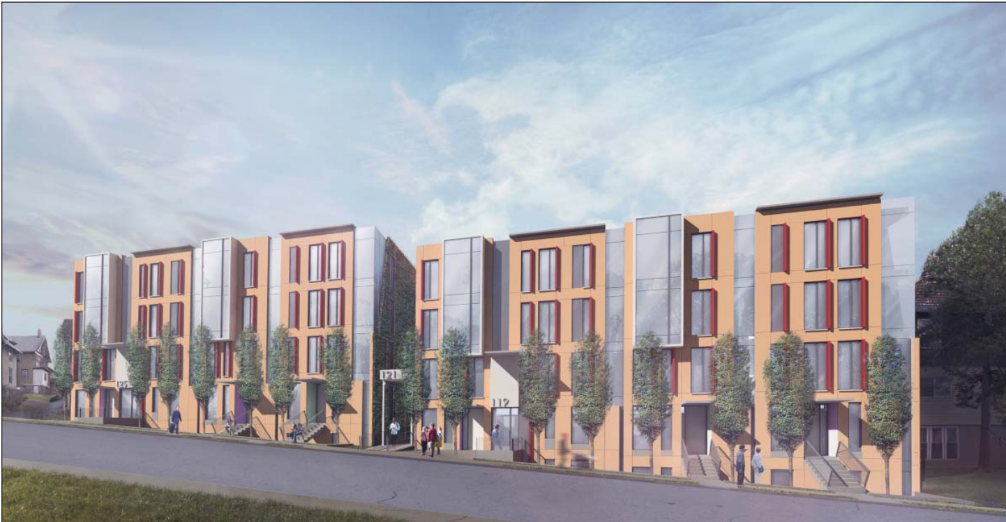
View looking northeast along College Avenue
